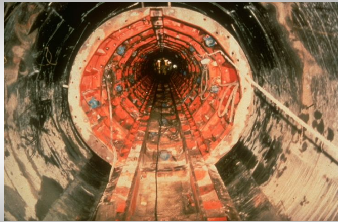
Stainless steel waterproof membrane in tunnel lining, Rovereto, Italy
