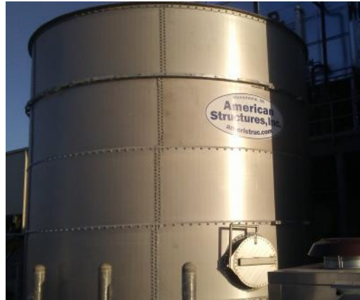
DMP Corp. — Mason, OH 18.46' x 17.33' EQ Tank 34,700 gal. storage capacity
