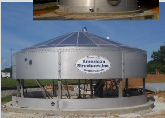
Rich Products— Morristown, TN (2 tanks) 1— 24.62' x 25' EQ Tank (80,600 gal. working capacity) 1— 27.69' x 25' EQ Tank (101,100 gal. working capacity)
